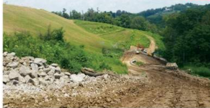
Embankment stabilization for pipeline project
