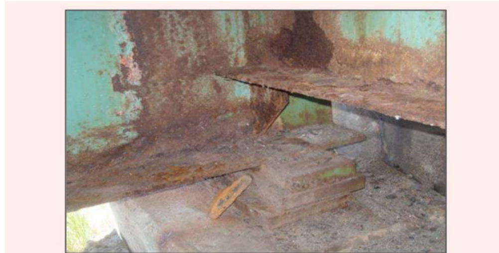
Figure 6 - Bearing Prior to Cleaning and Painting. Source MaineDOT.
