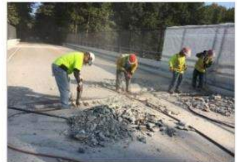
Eliminating a bridge joint prior to installation of link slab, Winch Ed over I-95, MD
