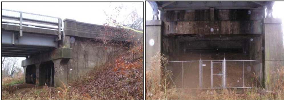
Photo 12 and 13: Bridge design mimicking “cave-like” atmosphere
