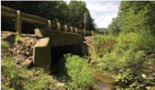
Existing and final downstream bridge of SR 46 over Pigeon Hollow Run.
