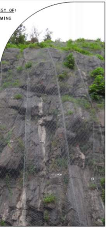
TYPICAL INSTALLATION OF ANCHORED WIRE MESH
