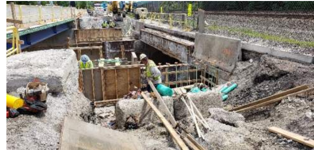
Construction of Second Phase Beam Seat Structure Girder on the Right
