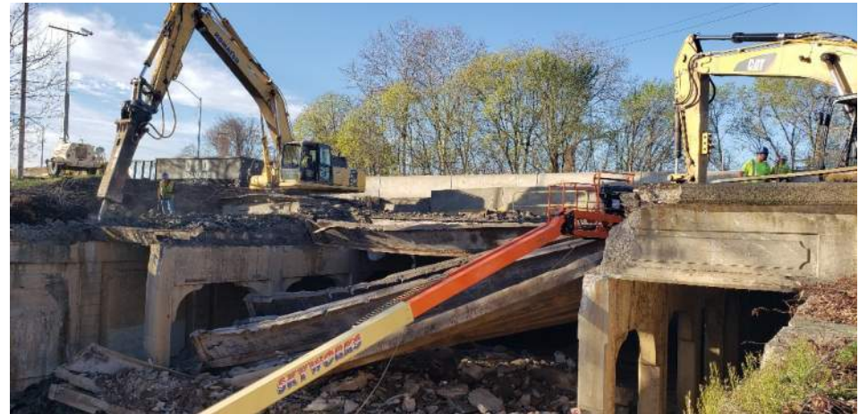
Demolition of First Phase
