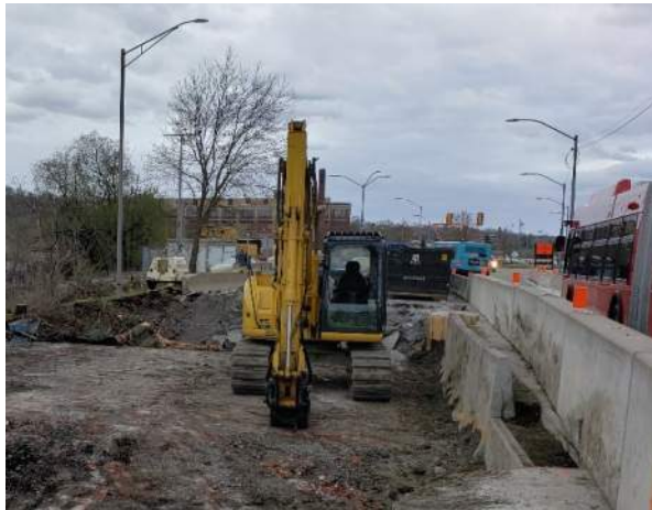
Excavation of Pavement and Subbase
