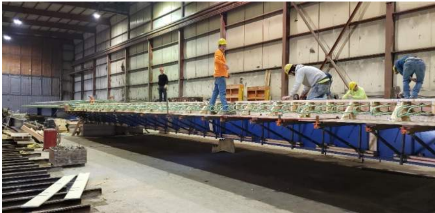
Module Casting Operations
