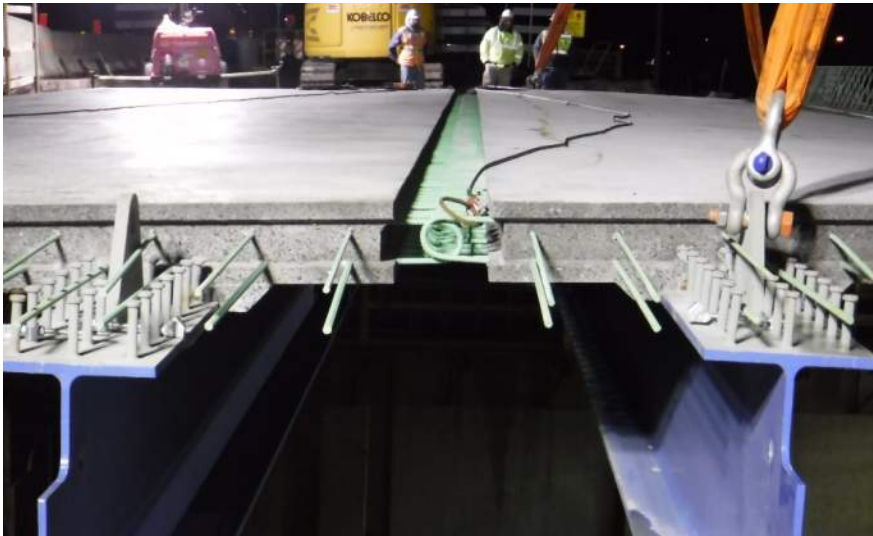
Typical Joint Between Modules
