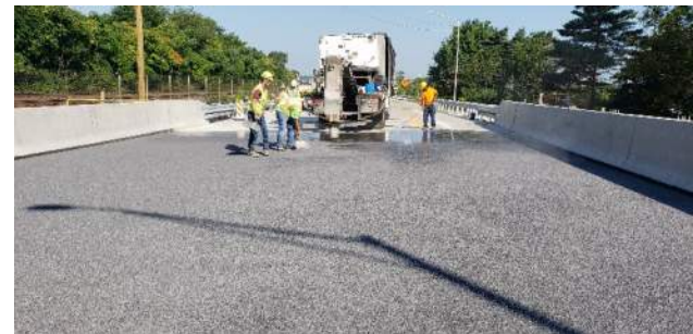
Application of Epoxy Overlay
