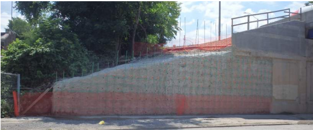
Existing Wingwall Jacketing
