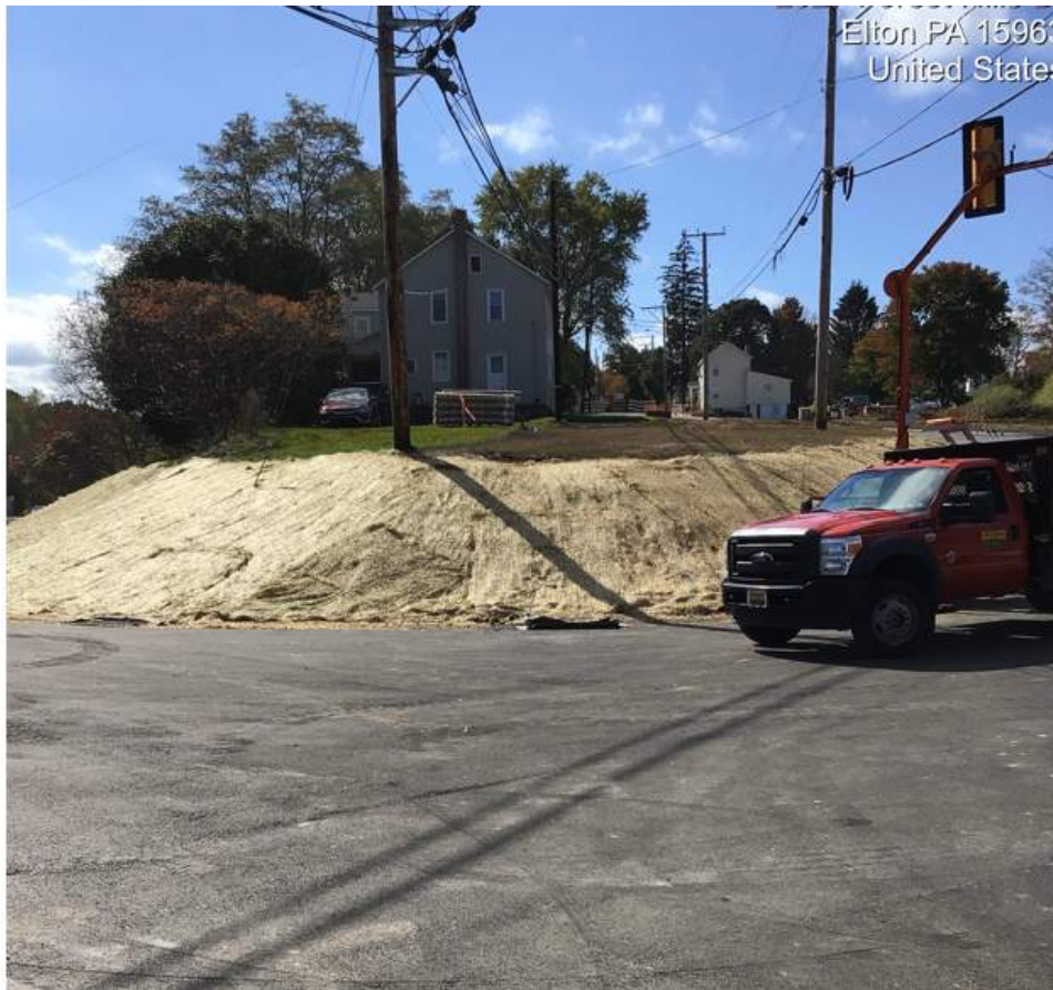
As designed cut slope with incorrect offset for determining ISD.
