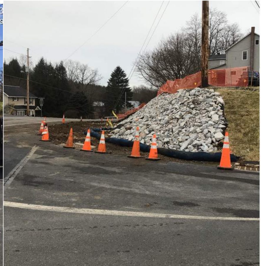
Slope corrected to increase sight distance.
