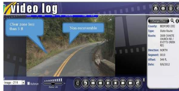
Figure A-8: Video Log for SR 3009, Segment 0010
