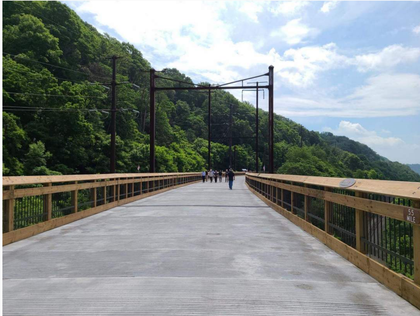
Safe Harbor Trestle Bridge
