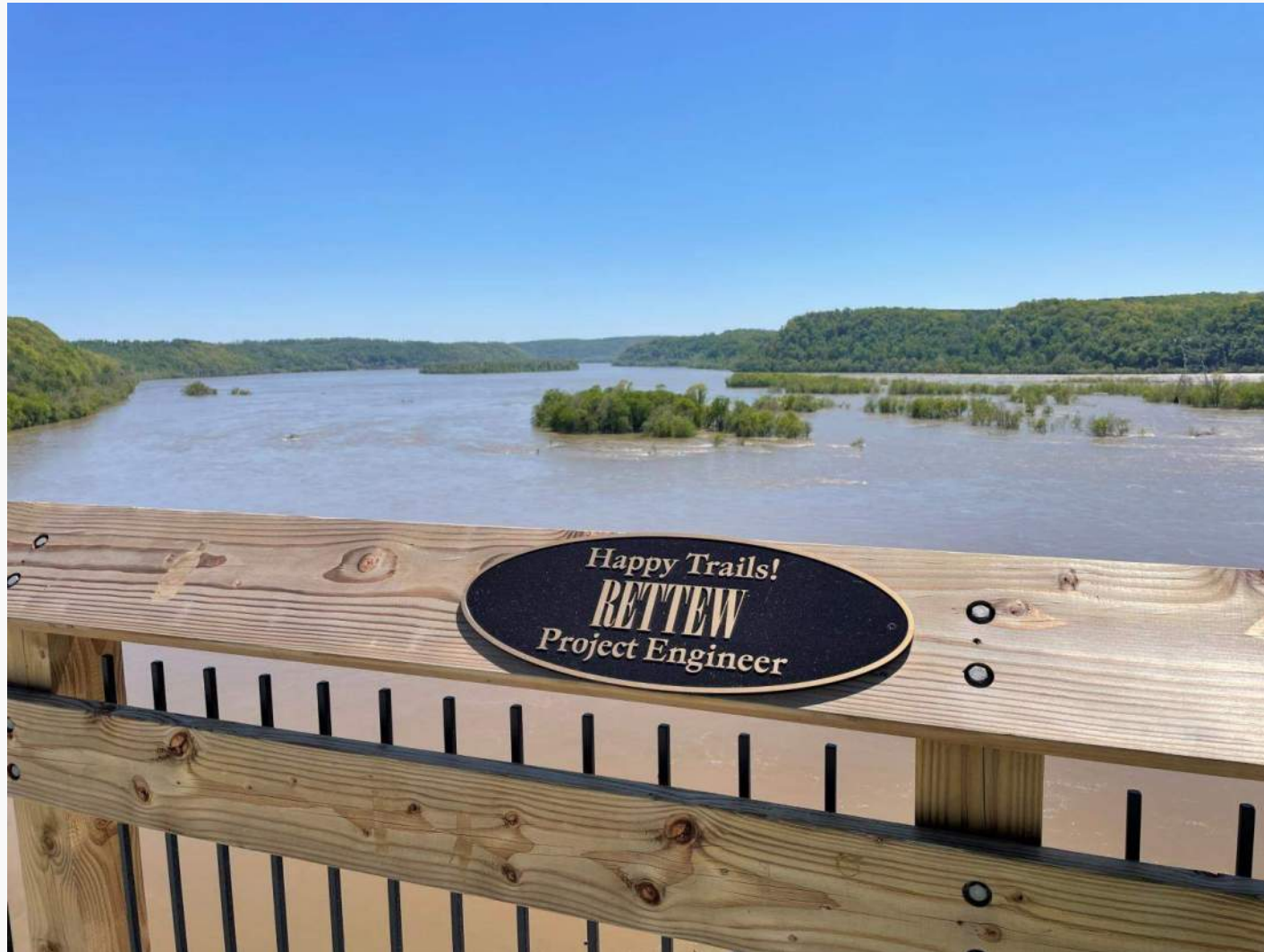
Safe Harbor Trestle Bridge
