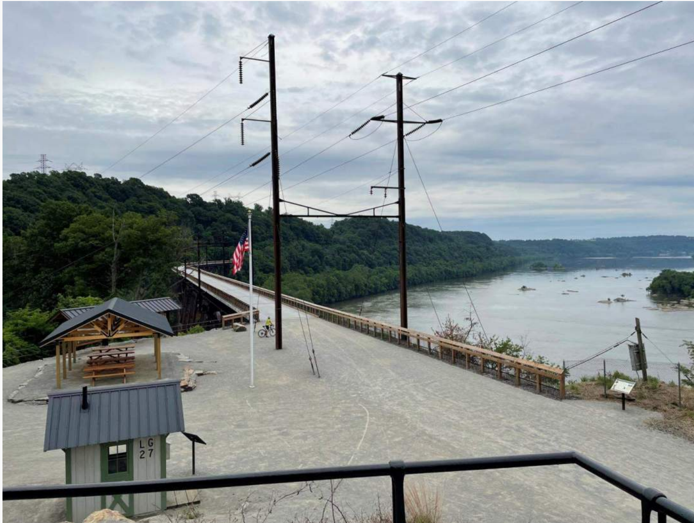
Safe Harbor Trestle Bridge
