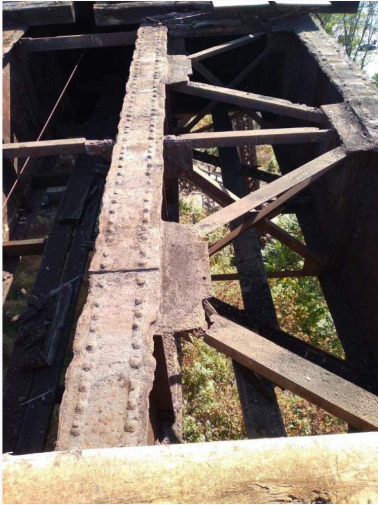
Safe Harbor Trestle Bridge
