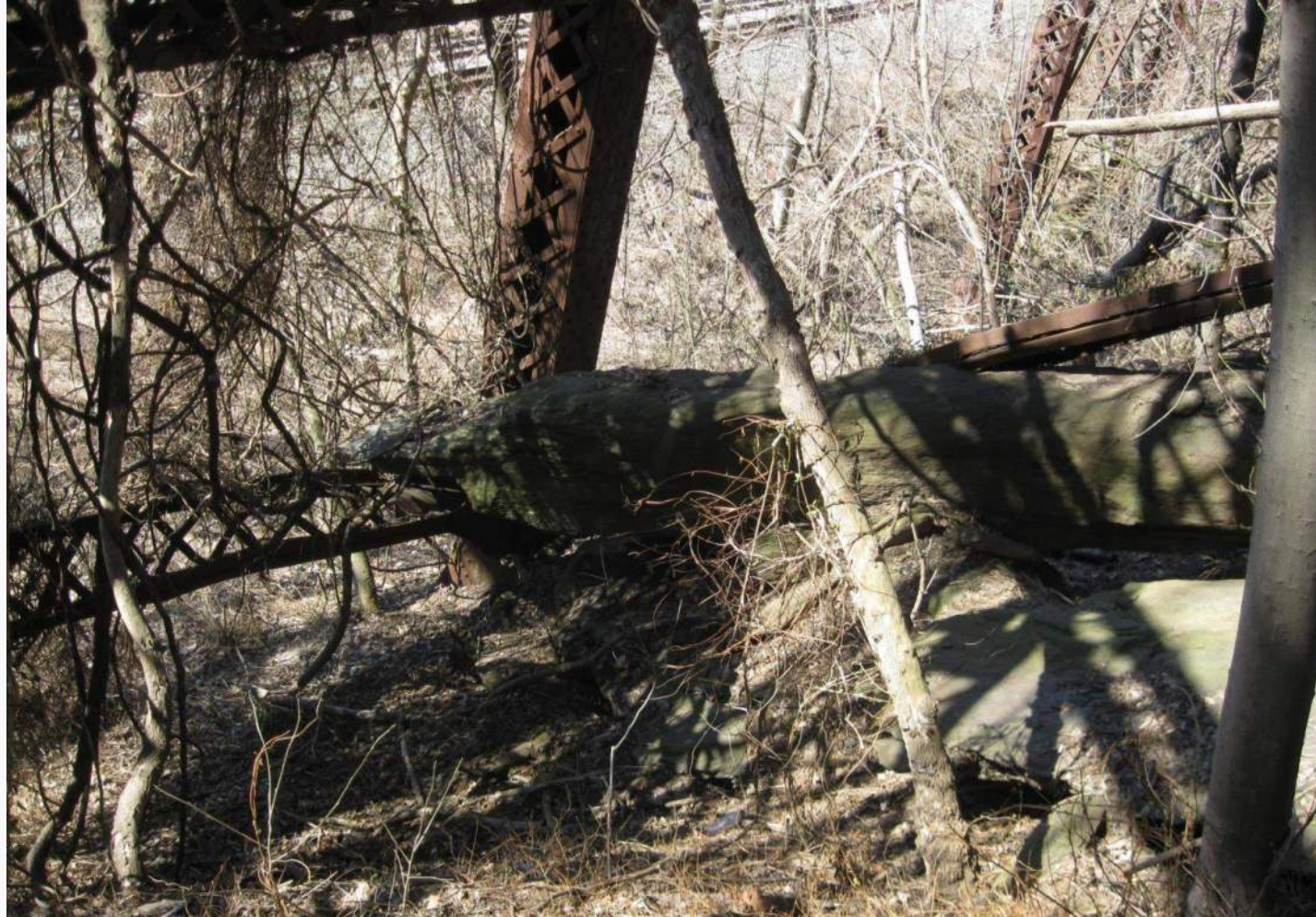
Safe Harbor Trestle Bridge
