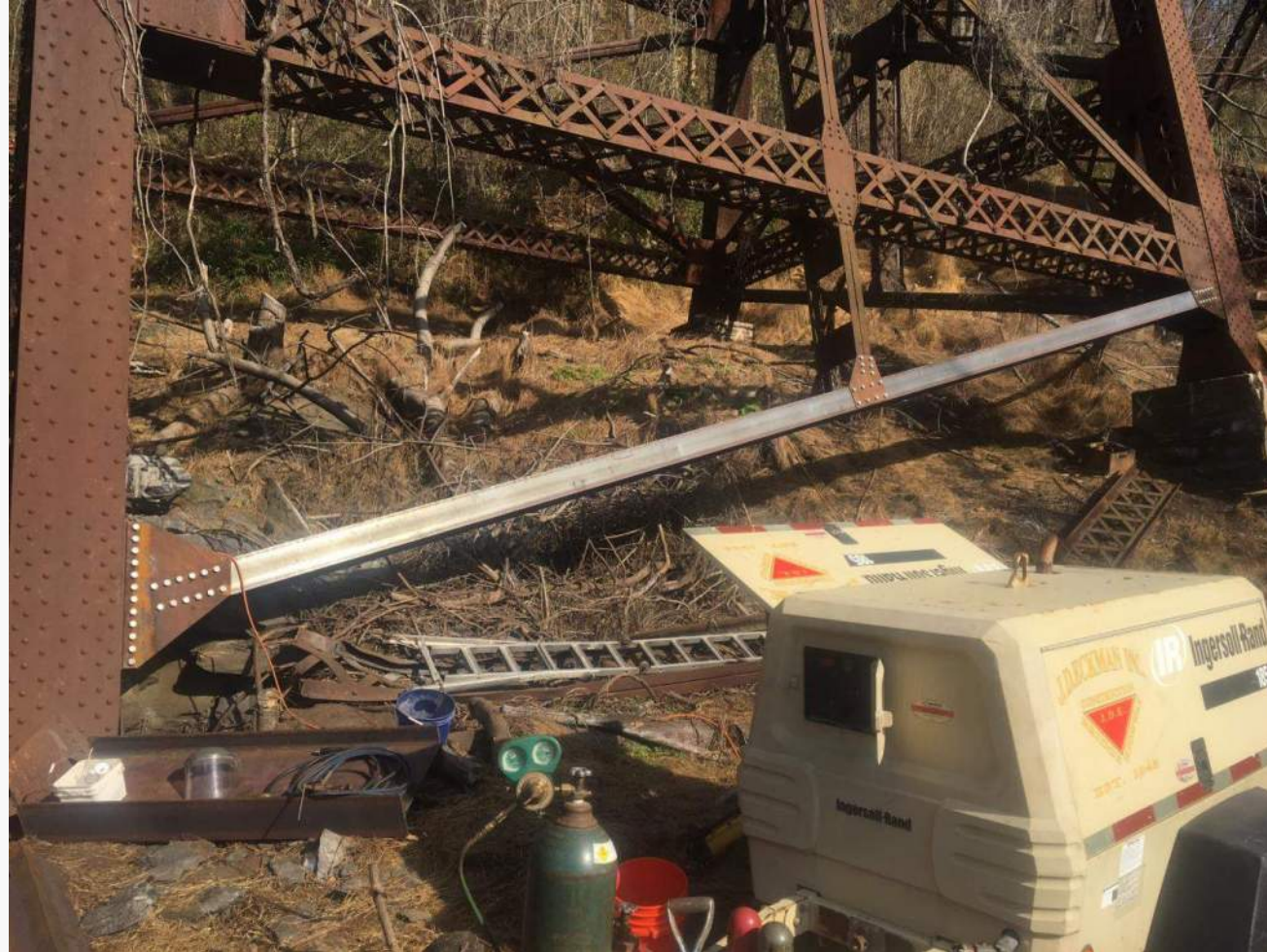
Safe Harbor Trestle Bridge
