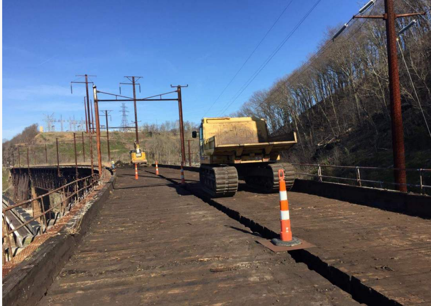
Safe Harbor Trestle Bridge
