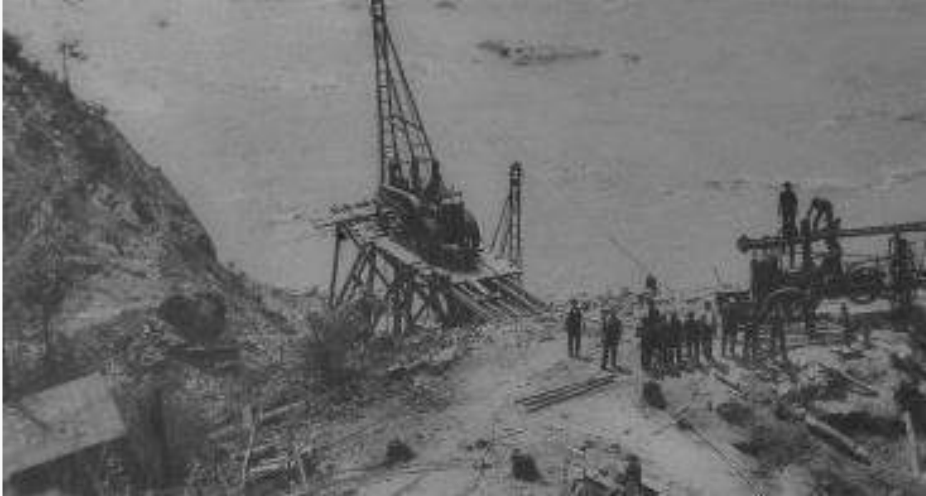
Safe Harbor Trestle Bridge
